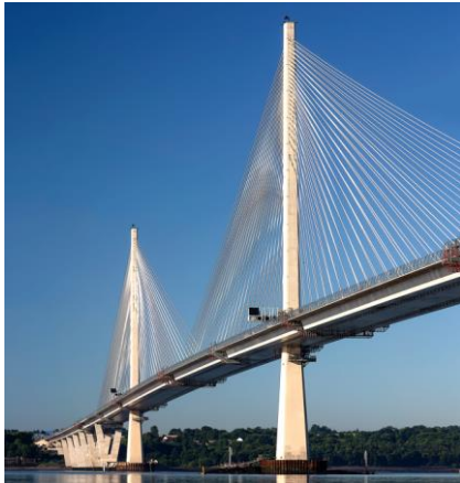
(a) Enkelt benet midterpylon (Queensferry Crossing i Skotland)
